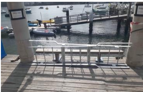
Stainless steel ladders waiting to be installed
